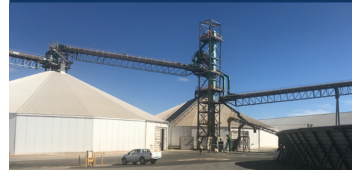
World-class grain producers group, WA Initiative to improve efficiency of port bulk storage and reception infrastructure. Challenge to modify rail due to land ownership, and existing conveyor systems unable to achieve targets.
